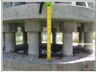
**Condition State 3**Anchor rod unsupported length above tolerance
