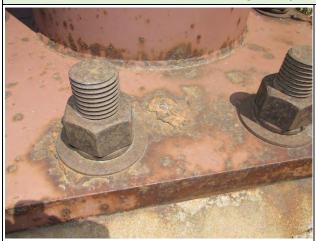
**Condition State 2**Corrosion initiated on base plate
