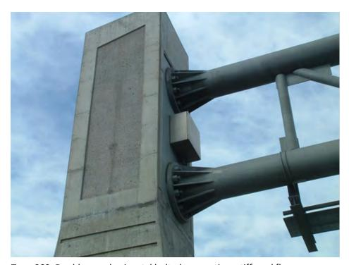
Type 060: Double arm, horizontal bolted connection, stiffened flanges
