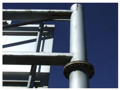
**Type 001:** Double arm frame, vertical bolted connection, welded to vertical pole
