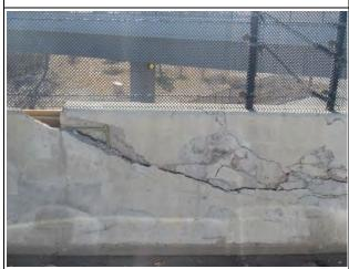
**Condition State 3**Spalls, delamination and exposed rebar
