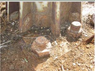
Corrosion with section loss on anchor rods, nuts, and washers
