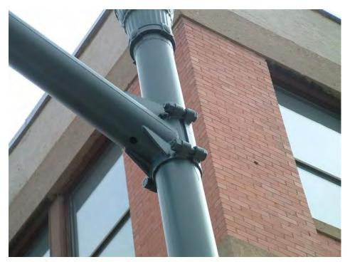
Type 117: Single arm, welded-clamped connection, with stiffeners
