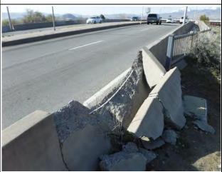
**Condition State 4**Severe Impact damage
