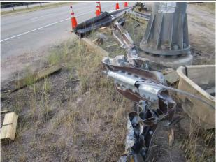
**Condition State 4**Severe impact damage to guardrail
