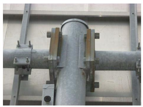
**Type 004:** Single face, single arm, double horizontal bolted connection to simplex plate
