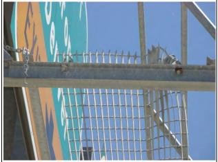
**Condition State 2** Minor impact damage to catwalk
