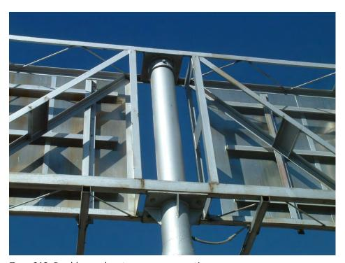
Type 019: Double arm box truss, cap connection
