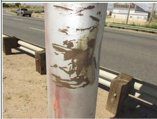
**Condition State 2**Minor impact damage
