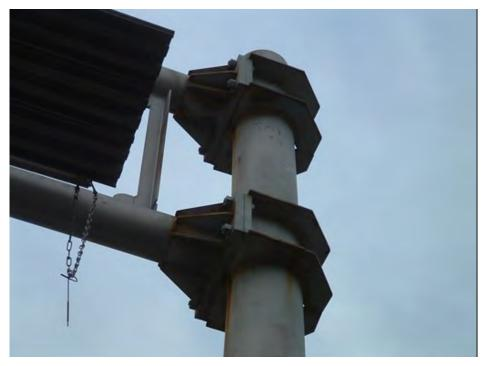
**Type 048:** Double arm, horizontal bolted connection to stiffener reinforced plates
