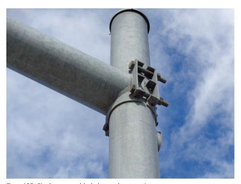
Type 105: Single arm, welded-clamped connection
