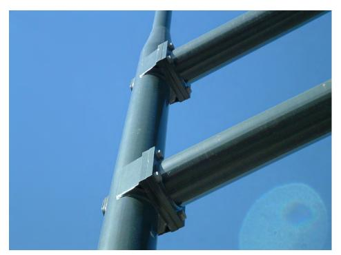
Type 114: Double arm, 4 bolt connection to simplex plate
