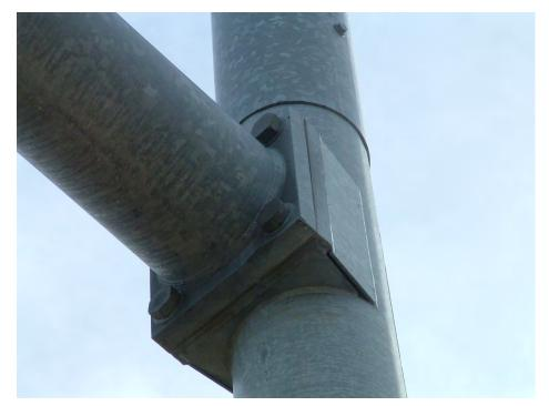
Type 100: Single arm, 4 bolt connection to simplex plate
