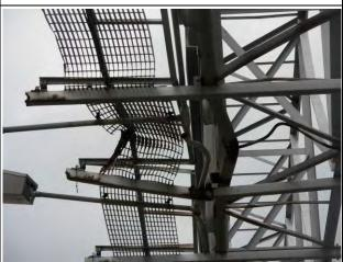
**Condition State 4**Damaged frame
