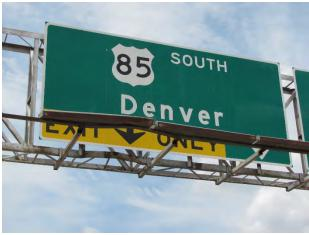
**Condition State 3**Impact damage to sign lighting
