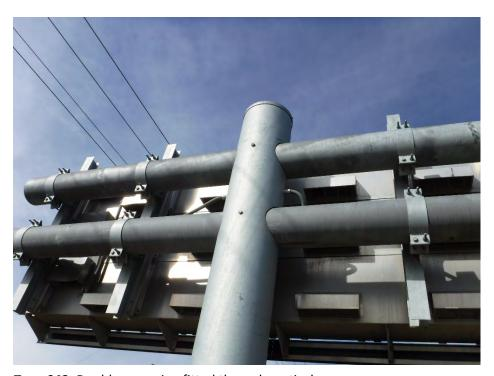
Type 042: Double arm, pipe fitted through vertical
