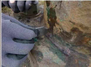
**Condition State 3**Corrosion with section loss of base weld
