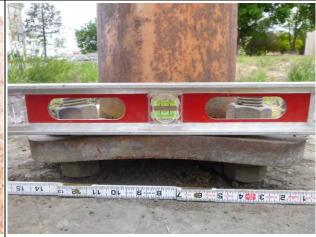
**Condition State 3**Distorted base plate
