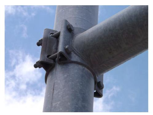
Type 112: Single arm, butterfly clamped connection
