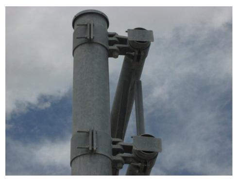
**Type 020:** Double arm, 5 finger collar connection, or 5 finger U-bolt clamp connection
