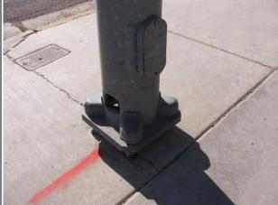
**Condition State 4**Punched hole in pole
