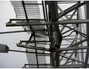
**Condition State 4** Severe impact damage to catwalk
