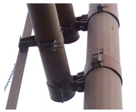
**Type 024:** Double arm, 6 finger collar connection, or 6 finger U-bolt clamp connection
