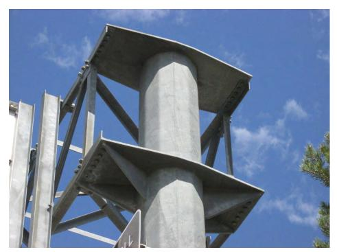
**Type 034:** Double arm (angle) truss bolted cap connection to plates welded to vertical
