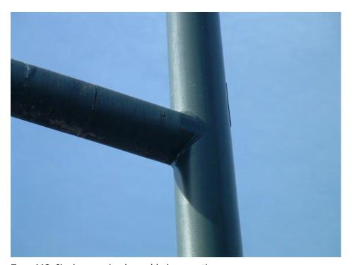
Type 113: Single arm, circular welded connection
