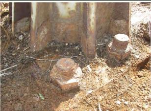
**Condition State 3**Corrosion with section loss on baseplate
