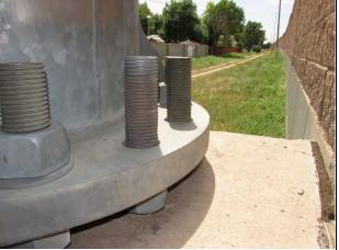
**Condition State 4**Missing anchor rod nuts and washers
