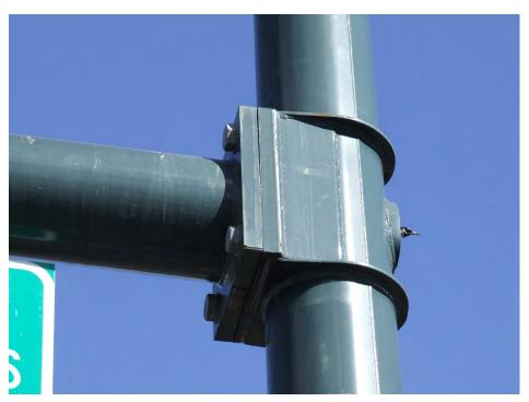
**Type 111:** Single arm, 4 bolt connection to simplex plate with welded bracket stiffener
