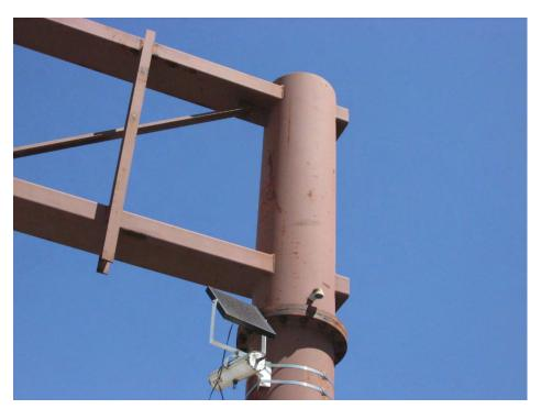
**Type 021:** Double arm welded through vertical, vertical bolted cap connection
