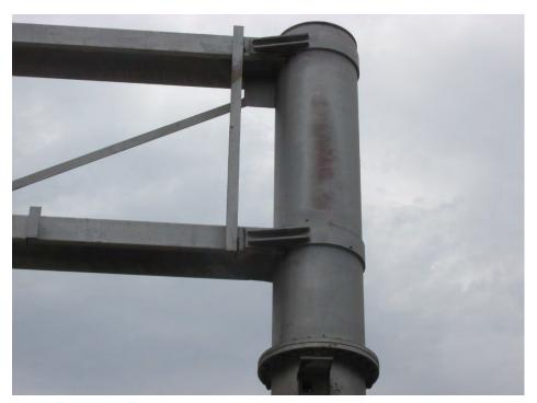
**Type 026:** Double arm, welded collar to vertical, vertical bolted cap connection
