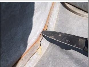
**Condition State 4** Fractured base weld
