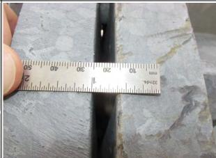
**Condition State 4**Gap in upper connection
