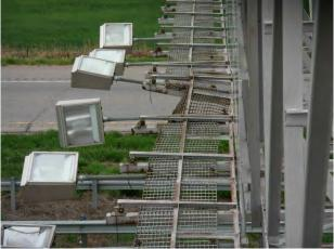
**Condition State 3**Lights damaged and not properly aligned
