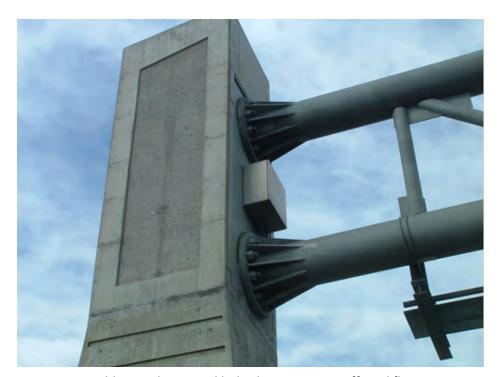
Type 060: Double arm, horizontal bolted connection, stiffened flanges
