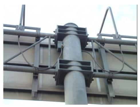
**Type 038:** Double arm, double horizontal bolted connection to simplex plate with welded stiffeners
