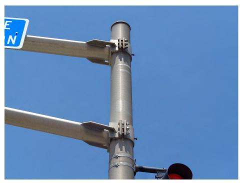
Type 110: Double arm, clamped connection
