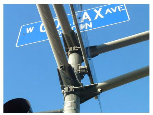
Type 109: Quad arm, clamped connection
