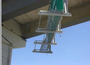
**Condition State 3** Impact damage and non-operational safety rail
