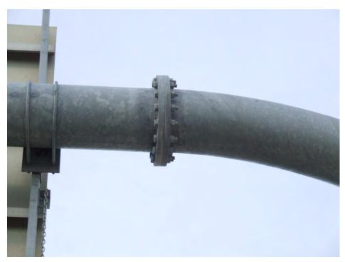
Type 006: Monotube, horizontal bolted connection, no stiffeners
