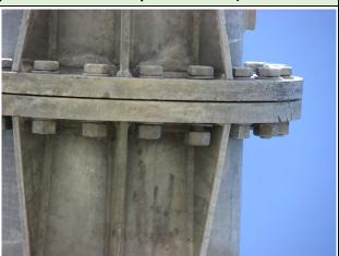
**Condition State 3**Loose nuts on upper connection
