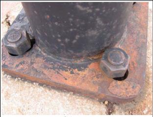
**Condition State 3**Oversized anchor bolt holes in base plate
