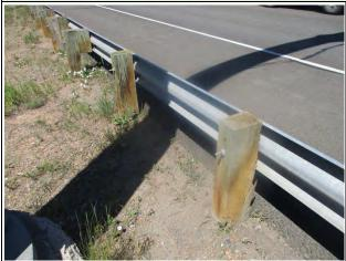
**Condition State 2**Missing blockouts at timber post
