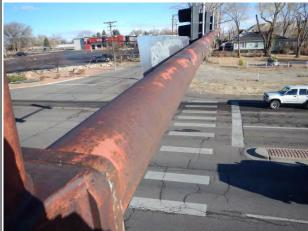
**Condition State 2**Corrosion initiated throughout mast arm
