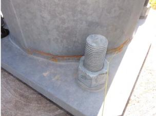
**Condition State 4**Fractured base weld protruding through steel pole
