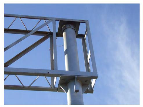
**Type 053:** Double arm (angle) truss, top cap connection, truss bearing on bottom
