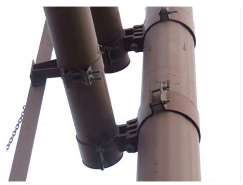
**Type 024:** Double arm, 6 finger collar connection, or 6 finger U-bolt clamp connection
